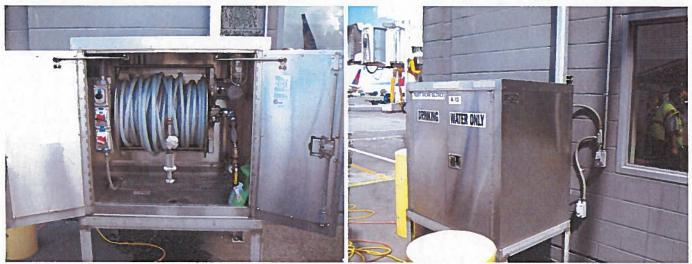
Airplane potable water filling station (Water Box) consists of flexible hose (200 feet) on a reel, backflow RP device, and control mechanisms.
